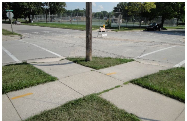
Perpendicular curb ramps aligned with crosswalks.
