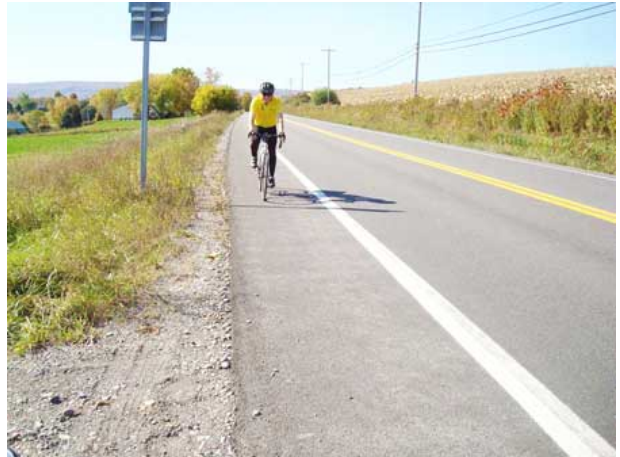
Paved shoulder. Source: Cornell Local Roads Program.
