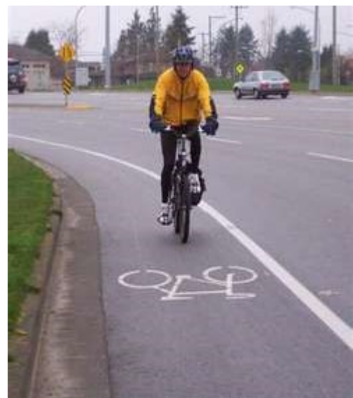
5' bike lanes provide sufficient room for cyclists to maneuver.
